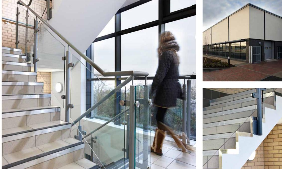
“ The CXT profiles are installed by double bedding the profile into the adhesive, which mechanically locks it into place, enabling specifiers to offer protection for ceramic tiles, whilst also providing building owners with peace of mind that the product offers superior protection from slips and falls. ”
